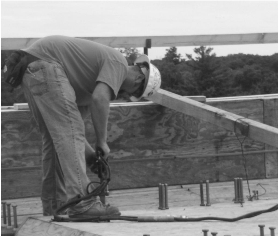
Figure 38. Posture maintained during traditional stud welding
