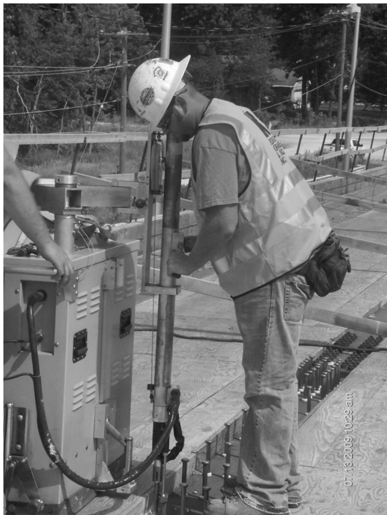
Figure 39. Posture maintained during stud welding with alternative system
